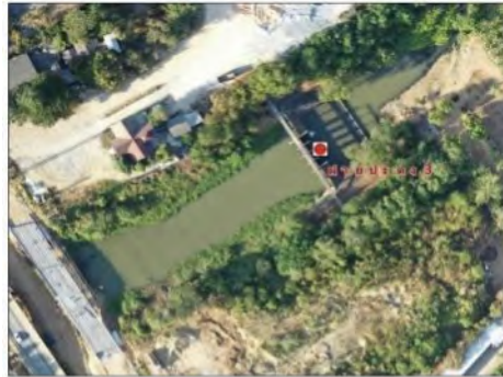
Reservoir Dam Structure Surveying
